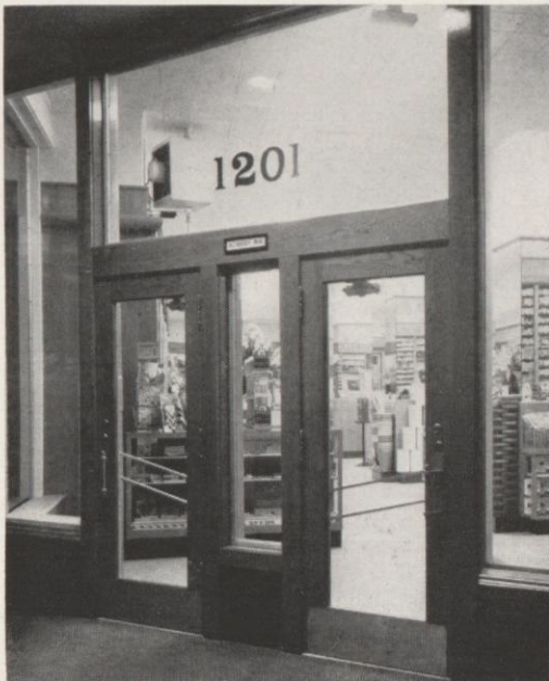
"High Vision" entrance and brilliant store lighting bring attractive store interior to the attention of all who are passing.
